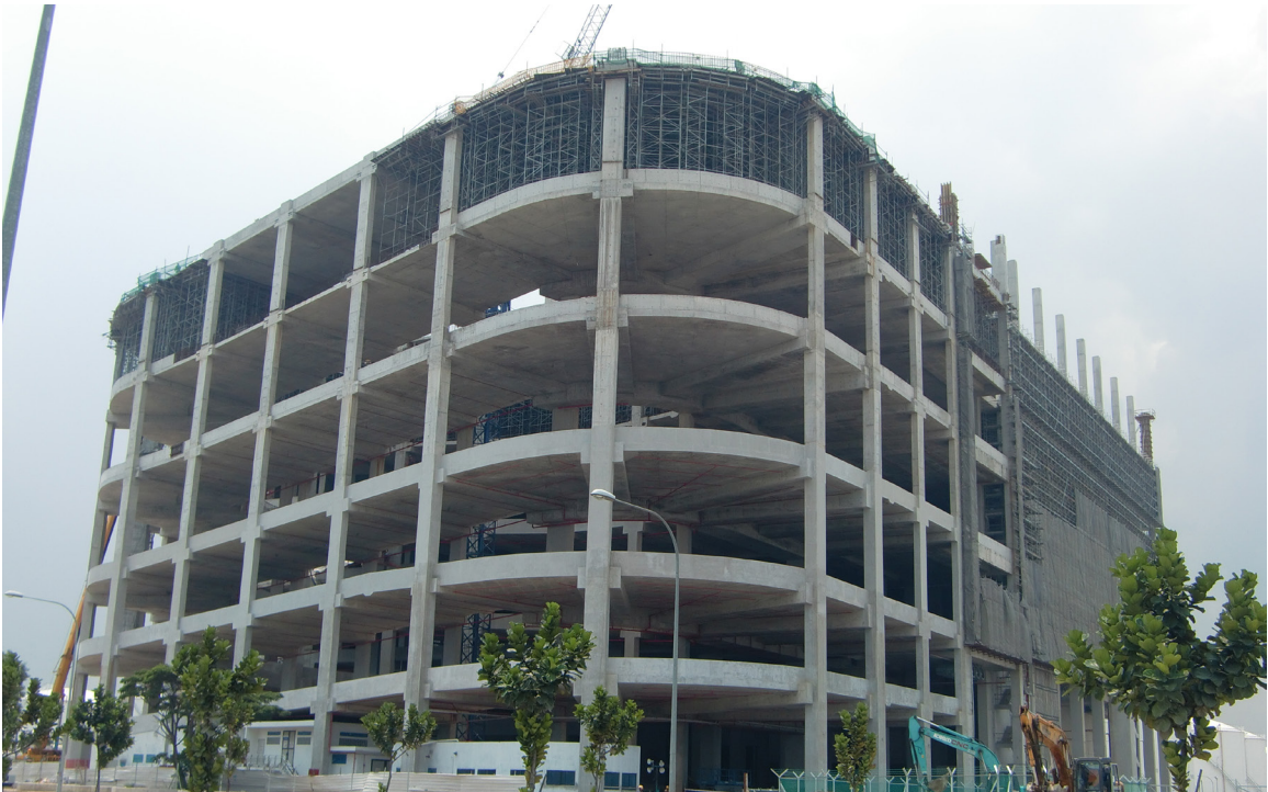
Vehicular Ramp @ Tanjong Kling
