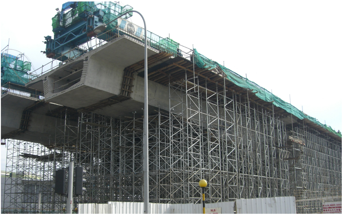
Viaduct Crossing @ Hougang Avenue 3
