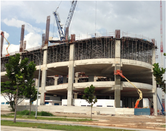
Vehicular Ramp @ Upper Changi Road
