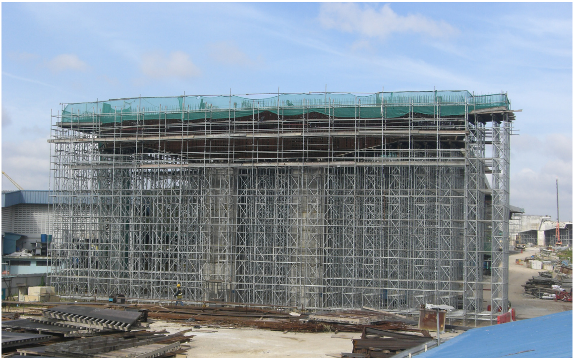
Pier @ Bartley Flyover
