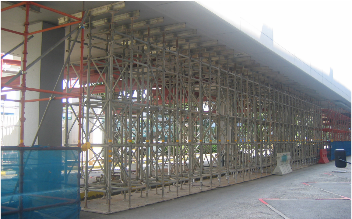
Viaduct @ People Mover System
