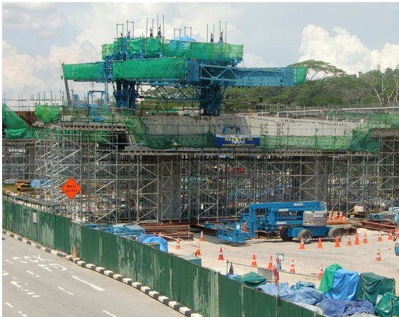
Pier @ Bukit Timah Flyover
