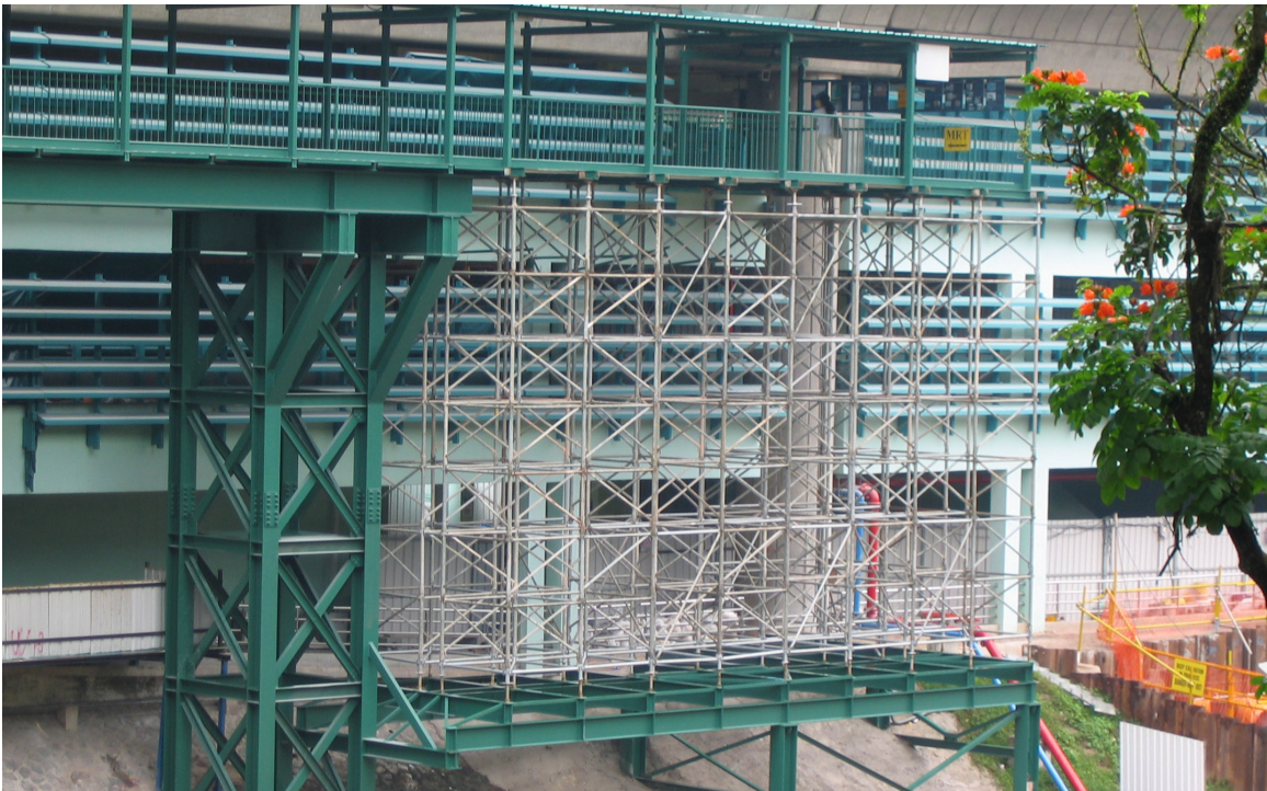
Pedestrian Bridge @ MRT Station
