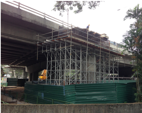
Pier @ Bukit Timah Flyover
